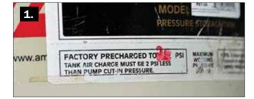
**1**—Accumulator tanks are typically pre-charged with a head of air (this one rated at 28 psi), which reduces the "water hammer" effect and pump short-cycling. **2**—Reliable selfpriming DC diaphragm pumps can eliminate the need for an accumulator tank in smaller systems. **3**—Larger vessels rely on 120 or 240VAC non-self-priming pumps. This model is equipped with a proprietary pre-filter to prevent debris from damaging the pump.
