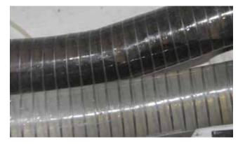
Potable-water systems, especially those with clear hose, are prone to contamination. The black accumulation inside the top hose doesn't bode well for the quality of the water that passes through it.
