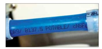
American Boat & Yacht Council (ABYC) and National Sanitation Foundation (NSF) standards for onboard potable-water systems require that all plumbing be approved to carry drinking water. The two examples of cross-linked polyethylene (PEX) tubing, **left**, carry either the "potable" or "NSF-61" designation, while the reinforced polyvinyl chloride (PVC), **below**, is labeled for potable water.
