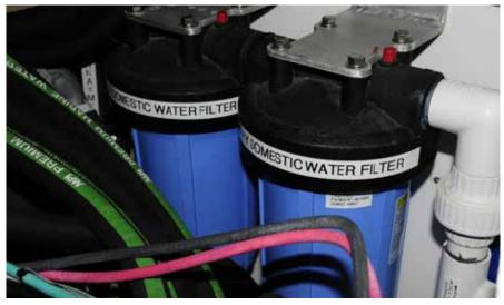
Whole-vessel filtration is gaining popularity as filters that can remove particulates as well as chlorine and heavy metals become readily available, inexpensive, and easy to replace.
